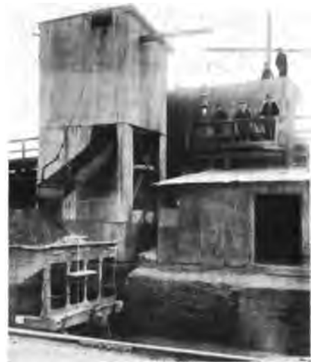
Fig. 2. Scene of Coal Crusher Accident.
